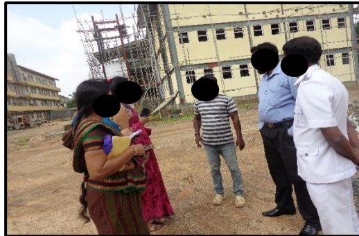
New building being built – Polonnaruwa Hospital
