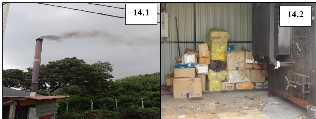
Incinerator at Trincomalee Hospital
